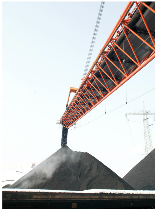
Coal-fired power plant in Scholven
